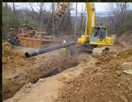
Installation of 18-inch pipe near the Prospect Reservoir.
