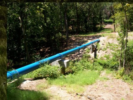
Completed 18-inch pipe across ravine.
