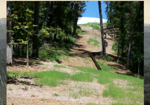
Revegetation of hillside with steep grades (25%) below the 3.5 million gallon Prospect Reservoir. All of the transmission line breaks occurred on this steep and undeveloped hillside.
