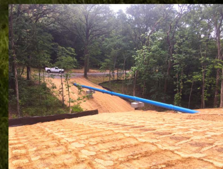
Ravine crossing following installation of erosion control matting.
