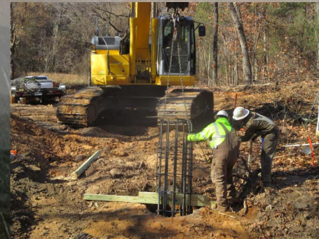
Construction of concrete piers for ravine crossing.
