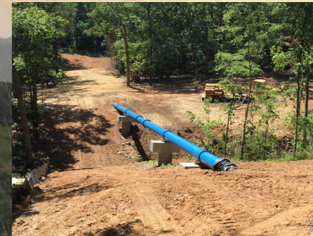
Completed ravine crossing prior to installation of erosion control matting.
