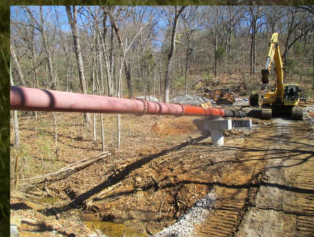
Installation of 18-inch long-span pipe.
