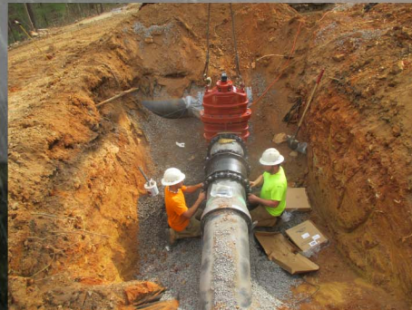
Installation of 18-inch isolation valve.
