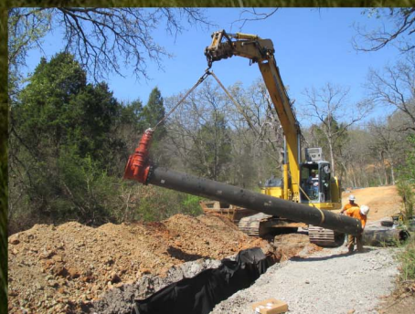
Installation of 18-inch pipe and gate valve.
