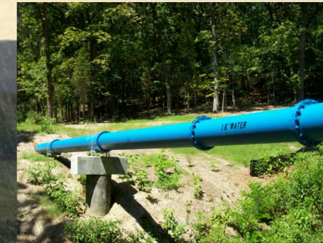
Completed 18-inch pipe across ravine.
