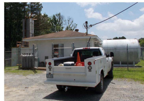
The water treatment plant was constructed in 1974. HW is currently designing a new state-of-the-art 1.0 MGD plant for the City.
