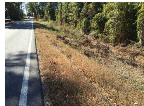
HW provided design phase services for the relocation of multiple water lines along U.S. Highway 335 in El Dorado, AR
