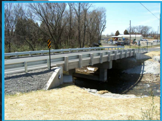
Pointer Trail East Bridge
