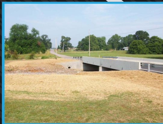
Richmond Road Bridge
