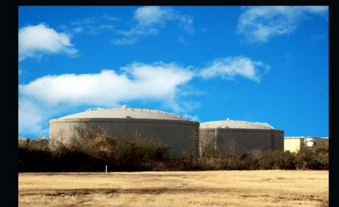
Zero Street Pump Station
