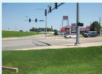
Project involved the relocation of multiple sanitary sewer mains along U.S. Highway 67/167
