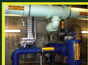
Design of the water treatment units and site piping include provisions to allow for the future expansion of plant treatment capacity to meet the 50-year peak daily water demand. The gravity filters may be modified from dual media to multimedia to increase their filtration loading rate and plant treatment capacity.
