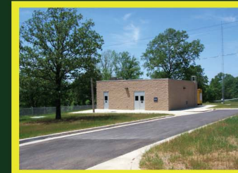
A finish water pump station was constructed at the plant to consolidate several independent pump stations in the water distribution system that were deficient in pump capacity. In addition to the new finish water pumps, the pump station also contains the filter backwash pumps.
