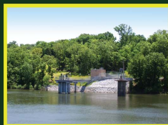
A raw water intake structure and pump station was constructed at Brushy Creek Lake, away from its south shoreline. This design approach borrowed construction techniques used in bridge construction, and was a cost savings measure.
