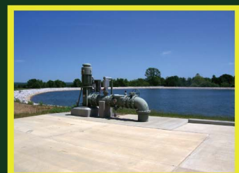
A finish water pump station was constructed at the plant to consolidate several independent pump stations in the water distribution system that were deficient in pump capacity. In addition to the new finish water pumps, the pump station also contains the filter backwash pumps.
