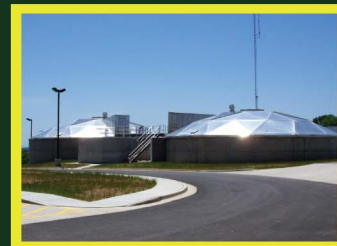
Design of the water treatment units and site piping include provisions to allow for the future expansion of plant treatment capacity to meet the 50-year peak daily water demand. The gravity filters may be modified from dual media to multimedia to increase their filtration loading rate and plant treatment capacity.
