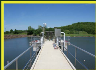
A raw water intake structure and pump station was constructed at Brushy Creek Lake, away from its south shoreline. This design approach borrowed construction techniques used in bridge construction, and was a cost savings measure.
